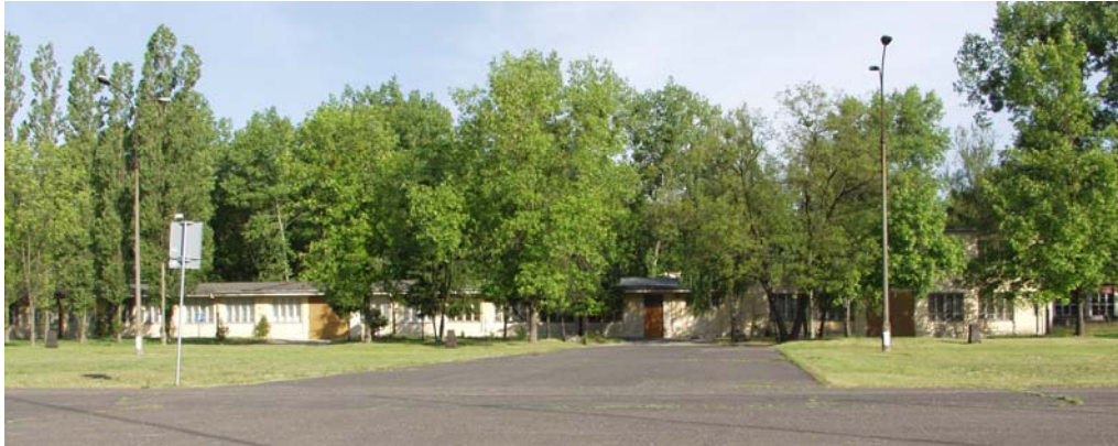
Picture 1. Building 69 –The Special Structure and Ballistics Section location
